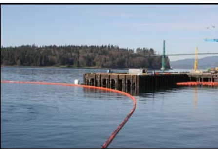
ContractorBoom deployed at oil shipping terminal
