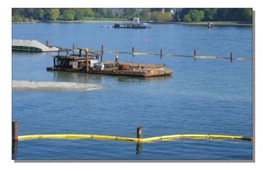
Canadyne **Silt Curtains** are floating barriers made of extremely durable high strength coated fabrics (impervious or pervious). Curtains incorporate foam filled floatation logs, and a fabric skirt with galvanized chain ballast in a fully enclosed pocket.
